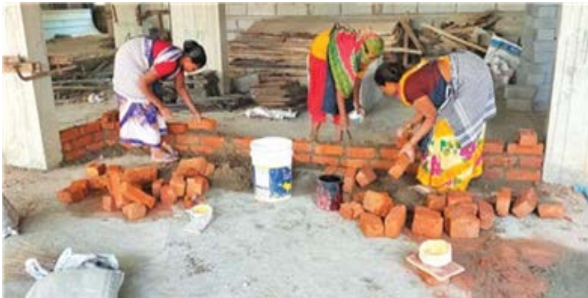
Fig 11: Women Construction Workers being trained to lay bricks on site
