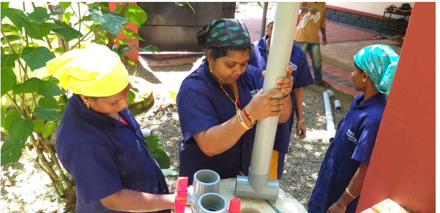
Fig 10: Plumbing and Well-recharging works being done by women construction workers trained
